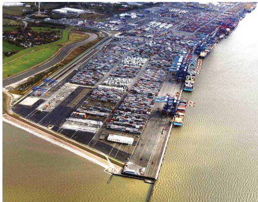
Fig. 6 ...and the finished terminal in 2008
