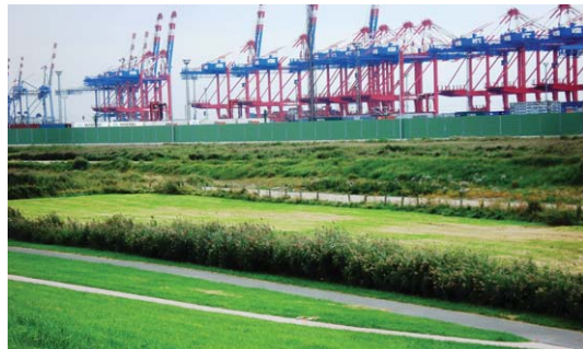
Fig. 7 View from dyke to the new Container Terminal 4
